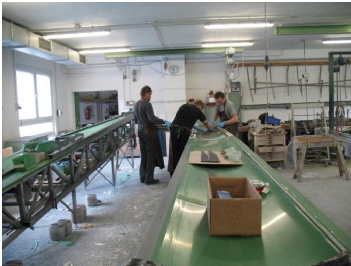
Getting some help with my pre-first-flight of the year (actually my ASG-29 wing being constructed at the Factory)
